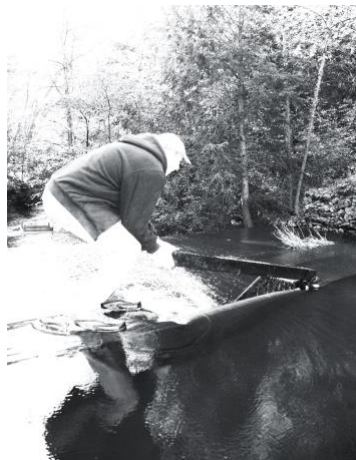
Fig. 3 Wangling a Spillway Board
