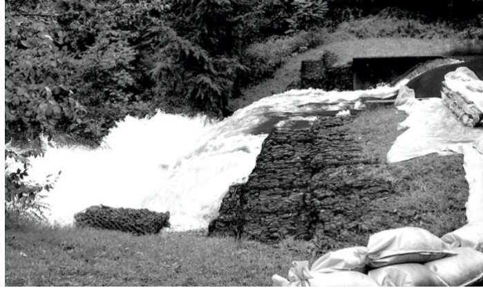
Fig. 1 Flood Waters Cascade Over the Dam in 2004
