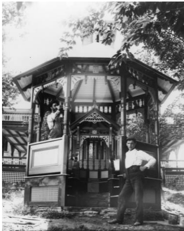
Fig. 3 Painters at Work ca. 1913
