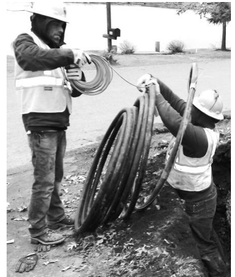
Fig. 2 Laying Line from Street to Pump
